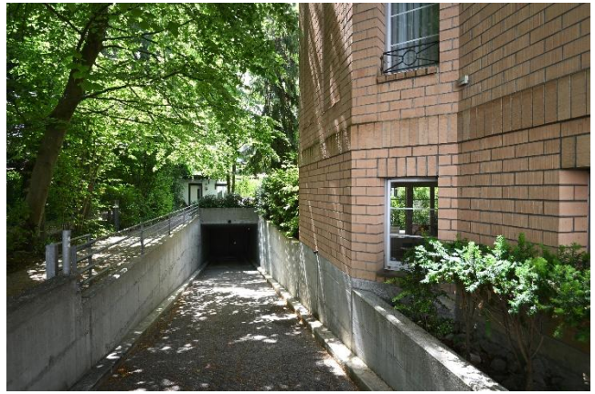
Driveway to the garage
